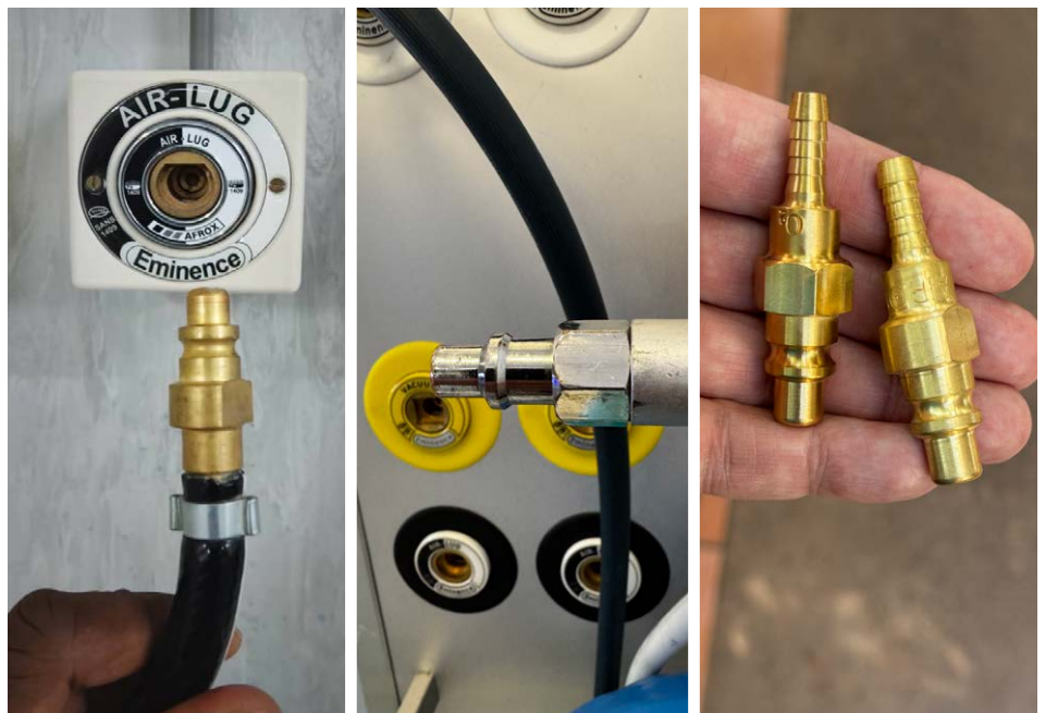
Fig. 22. High-pressure adapters (HPAs) for compressed air and oxygen: different standards often require change of adapters.
