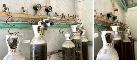
**Fig. 10.** Rundu State Hospital: central oxygen supply room with back-up oxygen cylinders.
